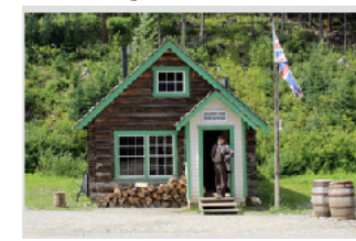
Williams Creek Schoolhouse
